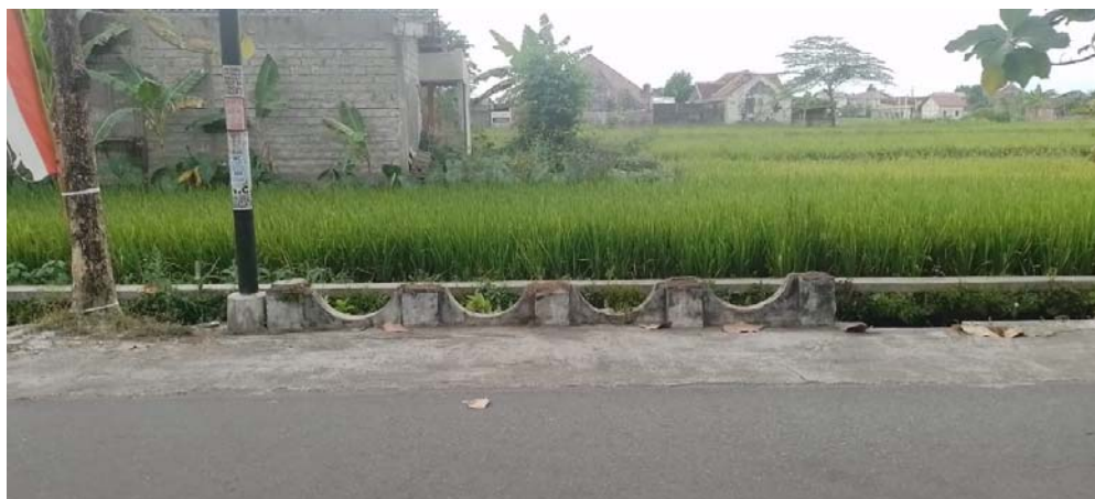
Figure 1. Location of the Flagpole Before being Repaired
