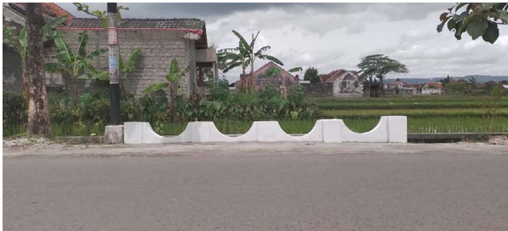
Figure 4. Place the Flagpole After Painting the Wall
