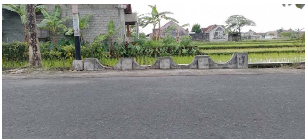
Figure 2. Location of the Flagpole After Repair
