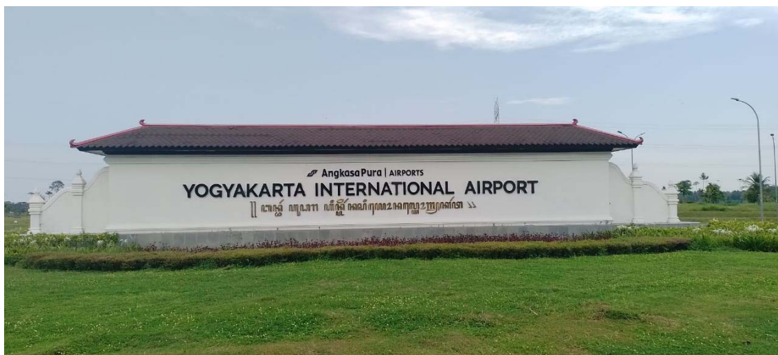
Figure 1. Yogyakarta International Airport
