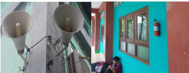
Figure 1. CCTV and APAR in every school building
