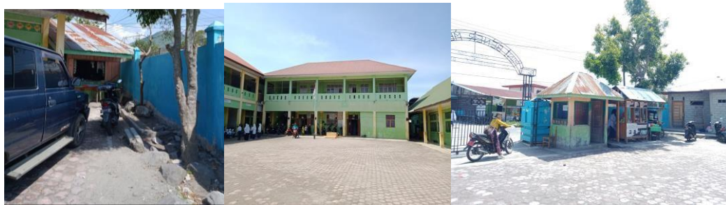
Figure 2. The condition of MIN 1 Bener Meriah's narrow field.
