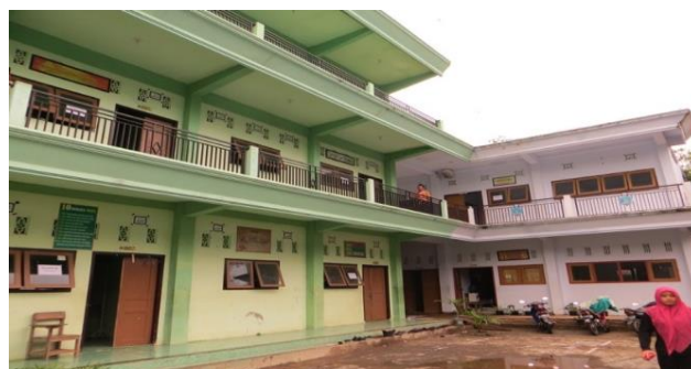
Figure 1. Environmental Conditions of SMKS Hudatul Muna 2 Ponorogo obtained by the author, through the condition of the yard, from the phenomenon of the scope it is reflected in the conducive level of school buildings (facilities).
